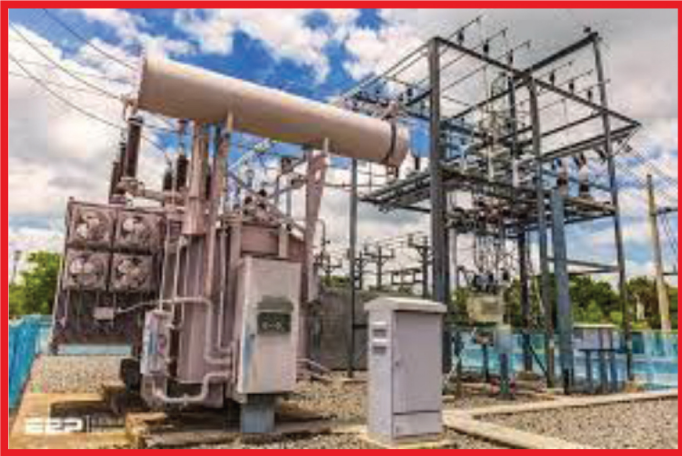
Construction of Sub-Stations and Switchyards
